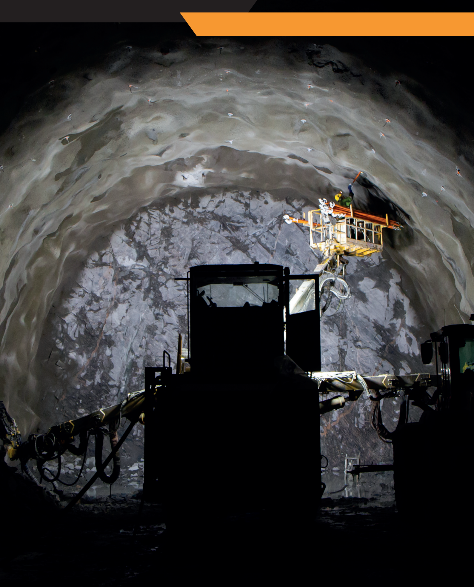
Rock support – M20 NC-Bolt Contractor: MossIA (Joint Venture Implenía Norge AS and Acciona Construction) Project: Railway tunnel, double track Sandbukta – Moss - Såstad, Norway
